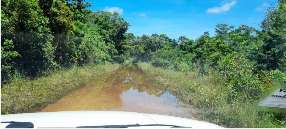
Figure 2: Inaccessible Road Boom Creek (Source: Ministry of Rural Transformation)
